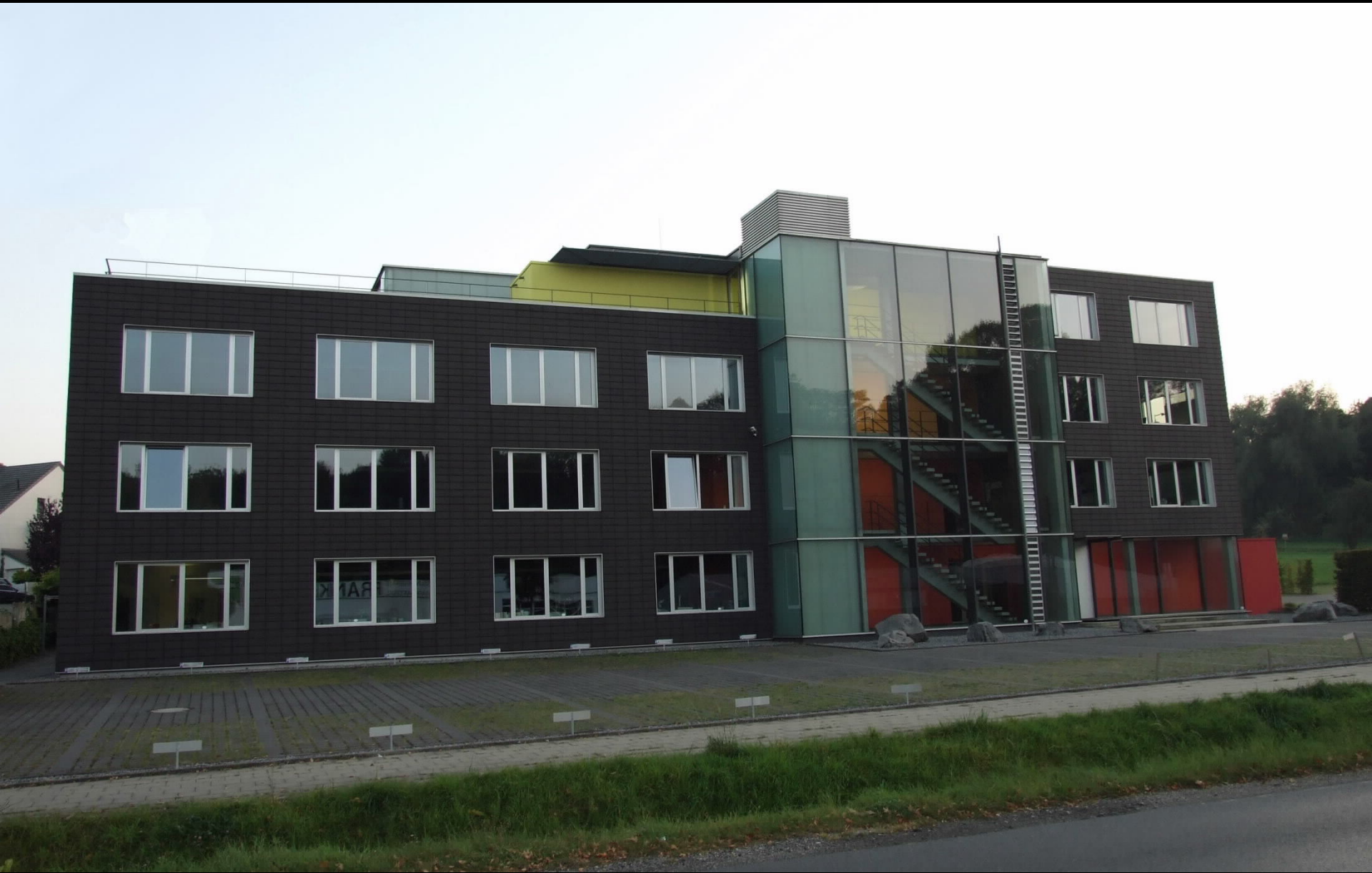
Photo: Aachen, Balanced Office Building, 2011, von Euku
